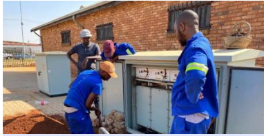
ELECTRICAL ENGINEERING | 6EP
